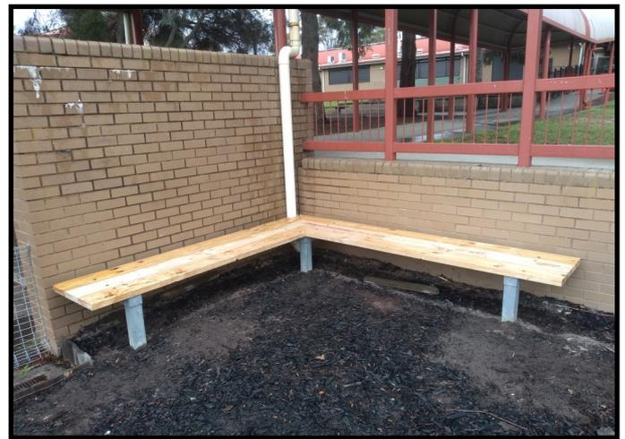
Constructing bench seating for the bottom garden area with recycled metal framework from the old seats on the "slab"
